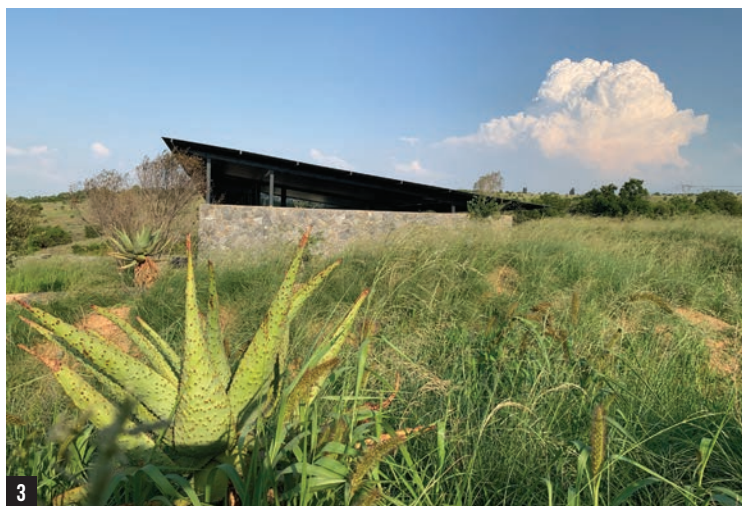
3 Western facade of the house which is clad in low-cost, recycled stone and submerged in the landscape to offer privacy from the street. 4 South-eastern view of the house "floating" over the landscape, illustrating the mono-pitch roof which is designed to enable passive cooling. 5 Exploded axonometric view illustrating the construction of the project. 1: Locally sourced stone walls. 2: Entrance walkway. 3: Steel roof structure. 4: Corrugated rood sheeting. 5: Indigenous trees in courtyards. 6: Cantilevered writing niche. 7: Corrugated sheet cladding. 8: Site anchored floating. 9: Steel framed structure. 10: Timber floors and timber decking.
